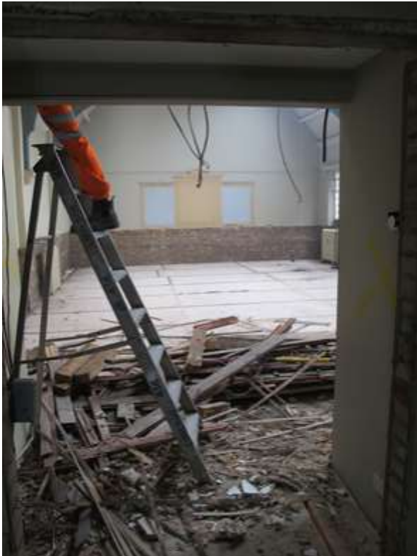
The Gibson Hall, with the kitchen wall removed.
