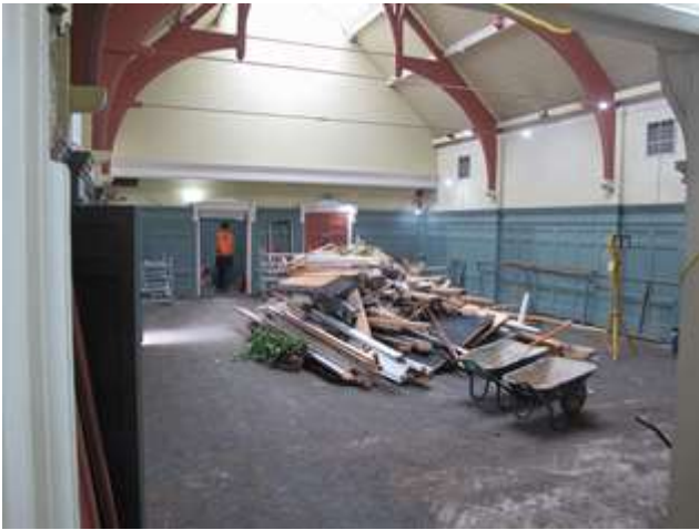
The St. Columba Hall, looking towards the lobby
