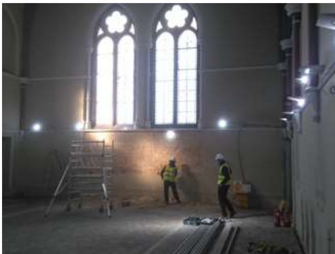
Preparing the wall of the sanctuary for the new windows on to Downing St.
