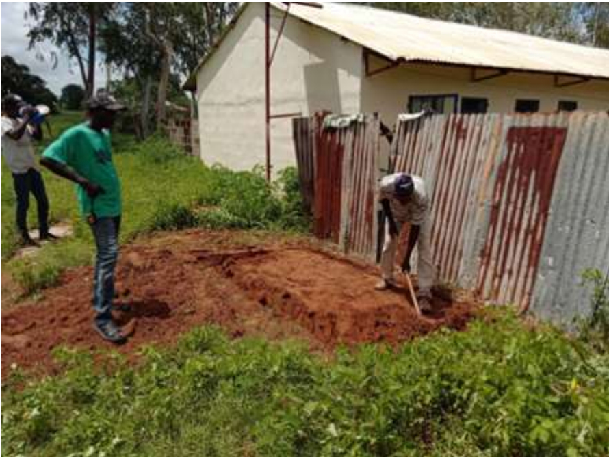
The foundations of the new toilet block currently being prepared.
