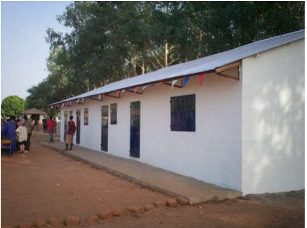
Teacher accommodation built with our support in 2008/9
