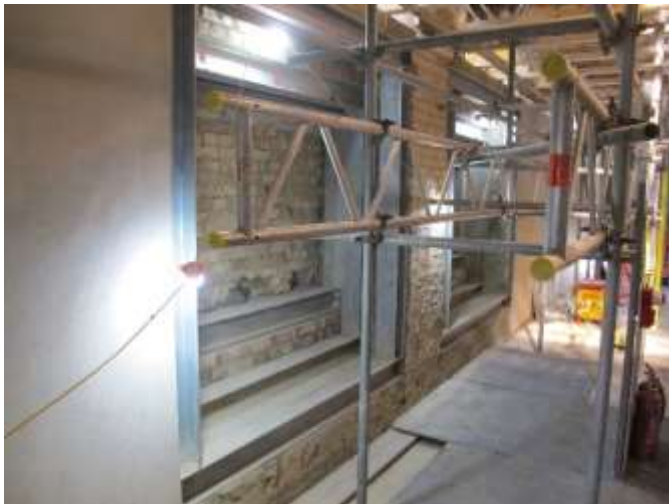
Steel frames ready for the new Downing Street windows
