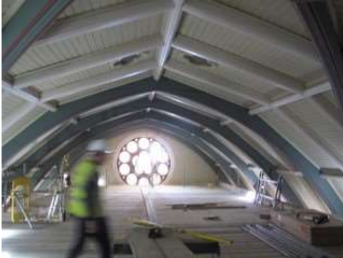
On the scaffolding “bridge” over the Sanctuary
