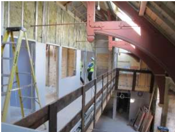
Hub – 1st Floor offices/rooms now formed
