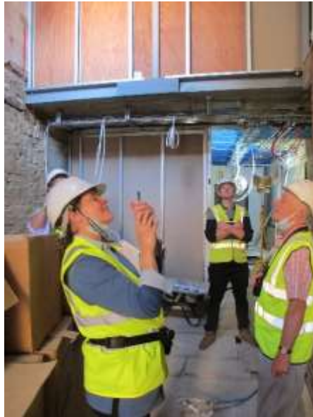
Viewing the space for the lift and main stairs
