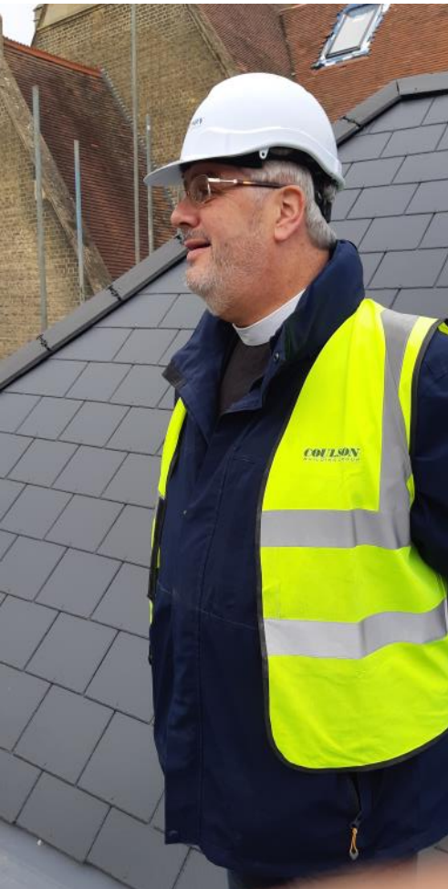
Nigel surveys the new roof
