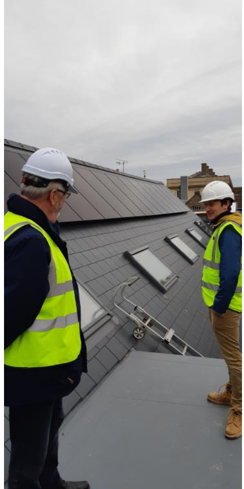
Nigel and Jack with the new roof lights
